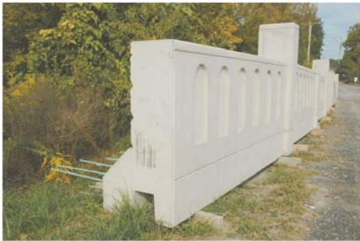
MSE WALL PANEL & PARAPET
