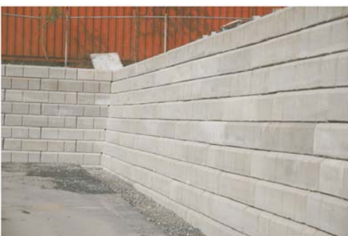
LARGE BLOCK RETAINING WALL
